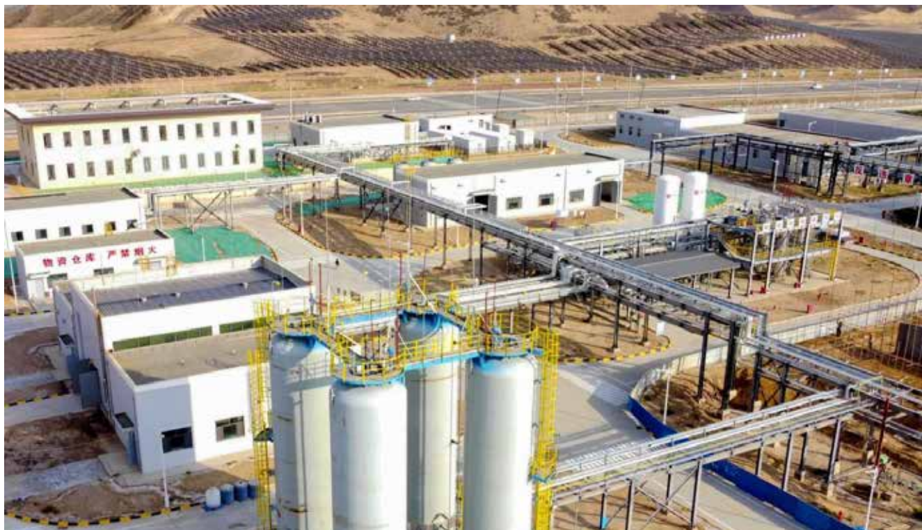
CO 2 Hydrogenation to Methanol "Liquid Sunshine" Project in Lanzhou, Gansu Province
