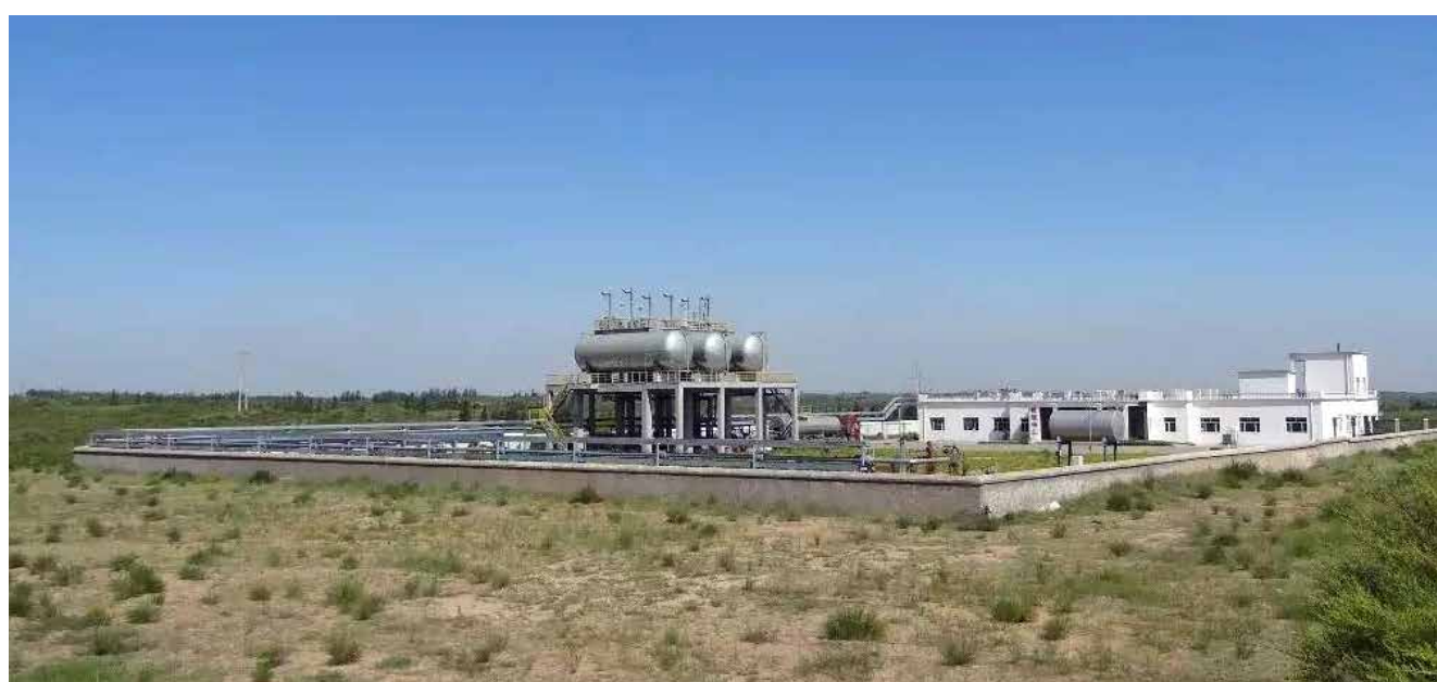
Shenhua carbon storage in saline aquifer project (Photo courtesy of Shenhua)
